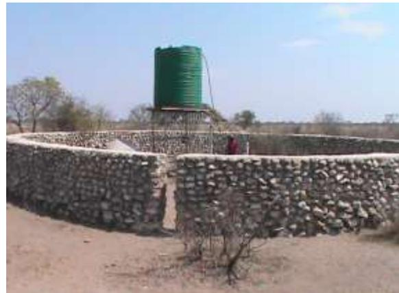
Figure 6.2 Water point wall protection
